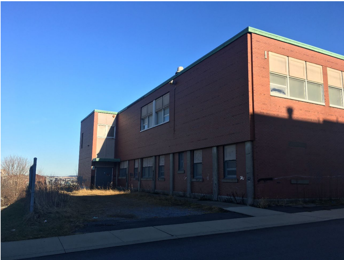
Subject site from City Line looking at the Northwest side of the site which abuts with property at 290 Tower Street
