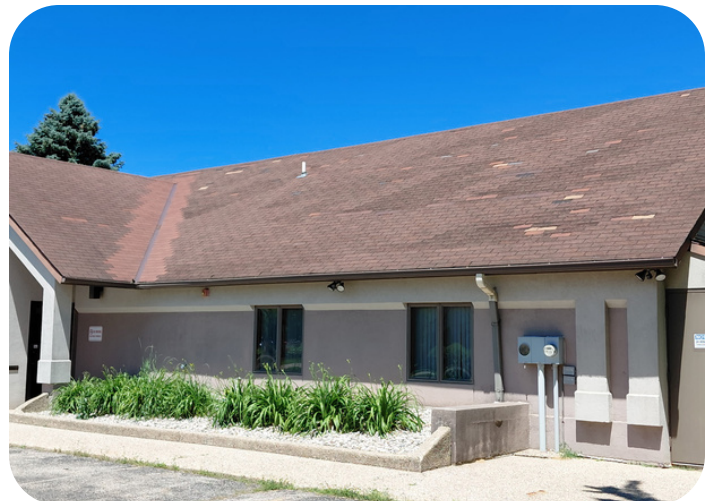
Replace Roof - Annex
