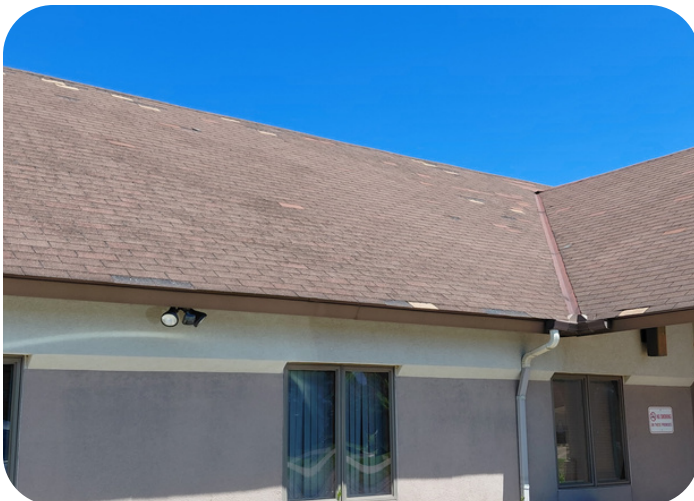
Replace Roof - Annex
