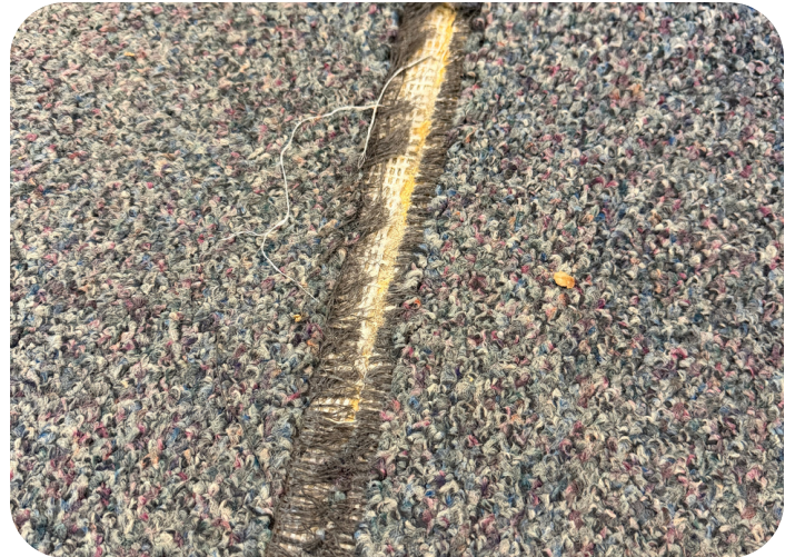
Replace Carpet - entire building
