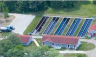
The McGowan Lake Hatchery, built in 1987, has helped to ensure the future of speckled trout fishing in western Nova Scotia, a region with many acid-stressed lakes and streams. This hatchery utilizes a unique water treatment facility to counteract the acidic nature (low pH) of the McGowan Lake water supply and an oxygen generation and injection system to rear nearly 1,000,000 Speckled trout which are released annually as fry, fall fingerlings and yearlings.
